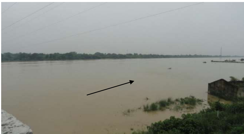
Figure 10.10 Rapti river downstream of NH29 (26.732984 N, 83.348470 E) - Left bank is elevated and right bank is flat, a bund is provided along right bank
