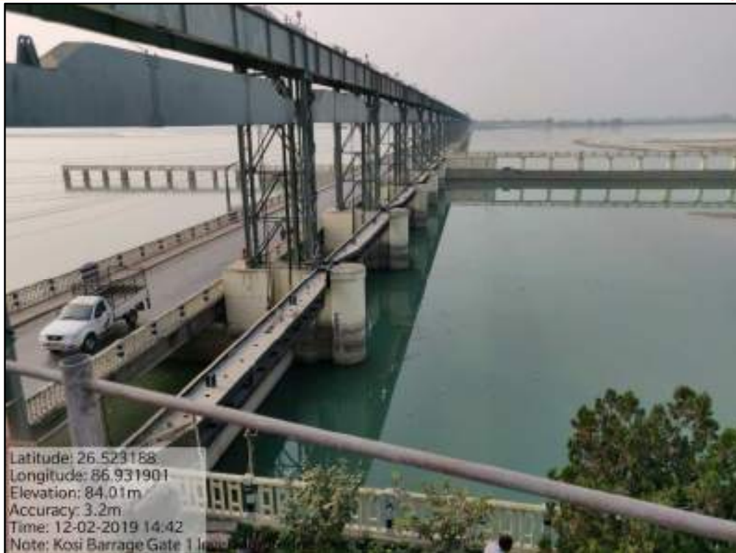
Figure 8-16: Kosi Barrage Gate System
