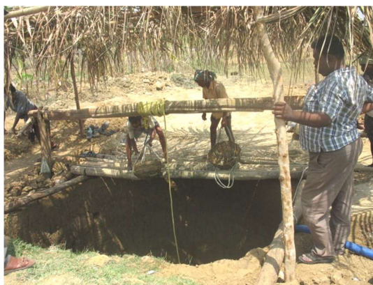
A view of the open well construction at the tail-end of right distributary under Madhyakhand sub-minor (2)
