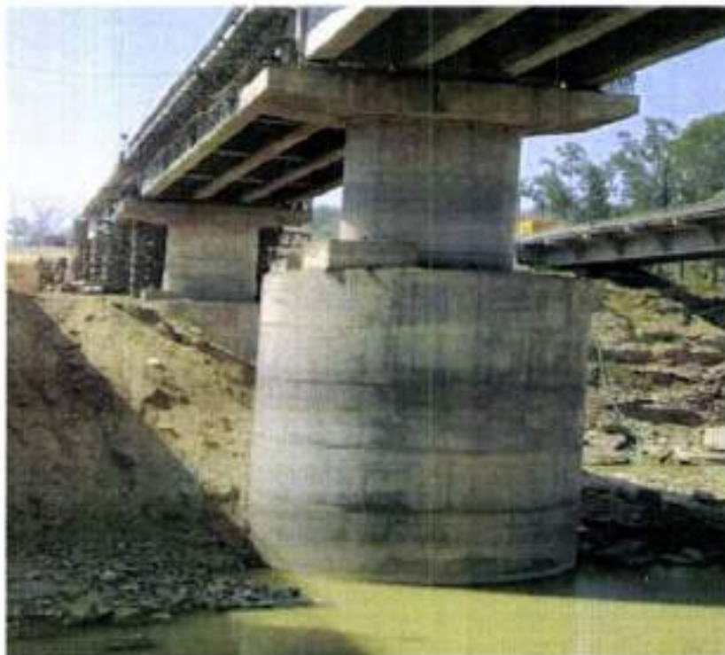
Fig. 1.2 Excessive scouring around footing of bridge on river Chakki, Punjab (Ramesh, 2012)
