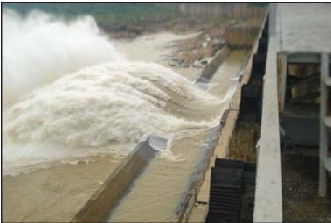
Rengali Dam showing Ski-jump Bucket and Hydraulic Jump
