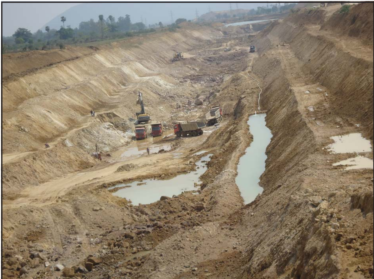
Excavation of RMC from RD.87 km to 89 km in progress
