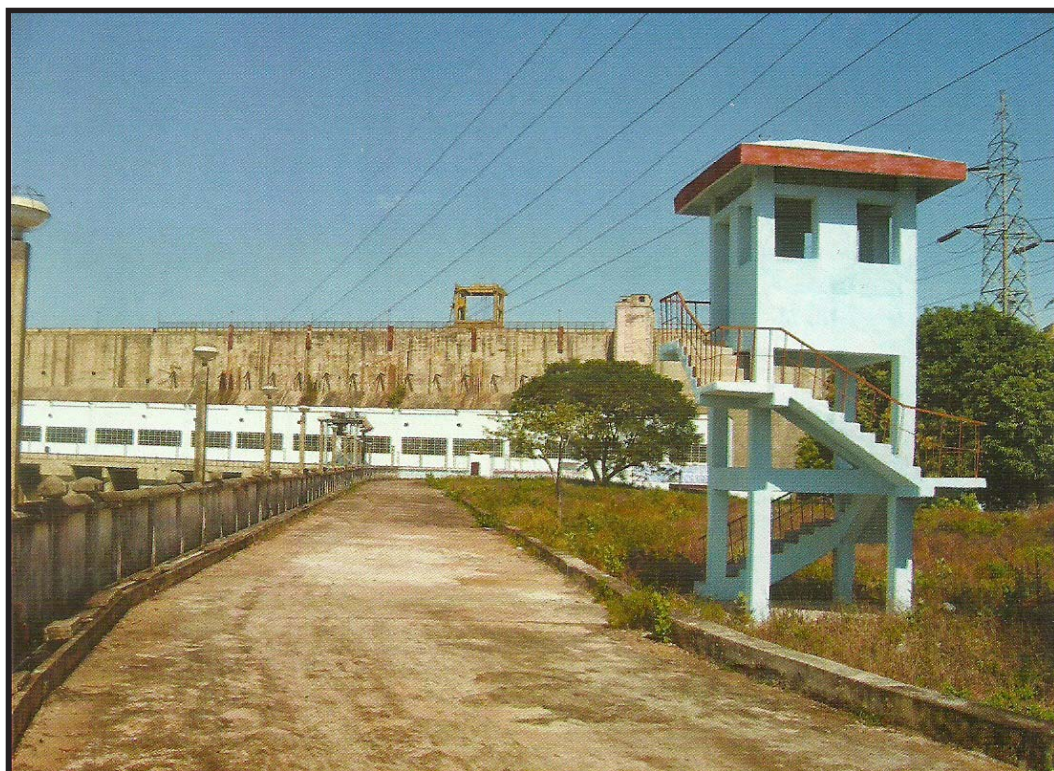
View of Rengali Power House
