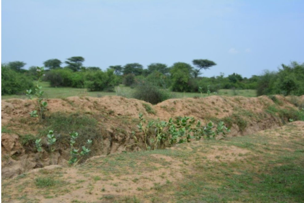
Figure 68: Mud barrier made by local people in between the drainage path
