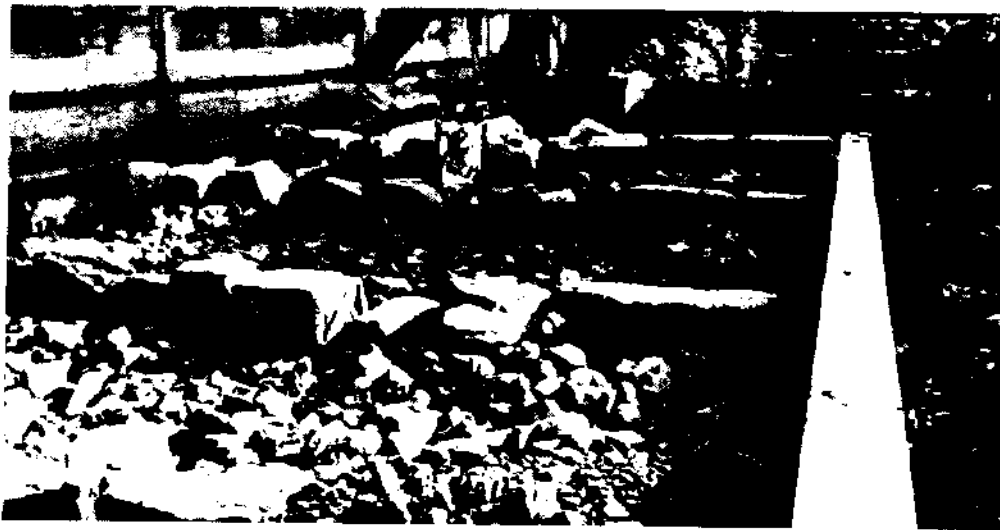
Fig.2.9 Crossbar block ramp application in the Wupperriver, Germany (Oertel and Schlenkhoff, 2012)
