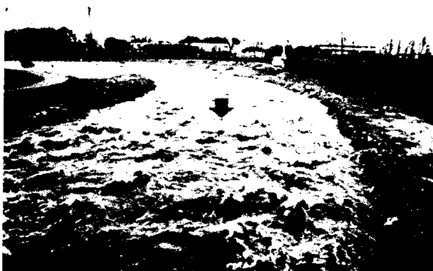
Fig.2.14 Undulating or tumbling flow conditions in an unstructured block ramp application on Wyna River, Switzerland
