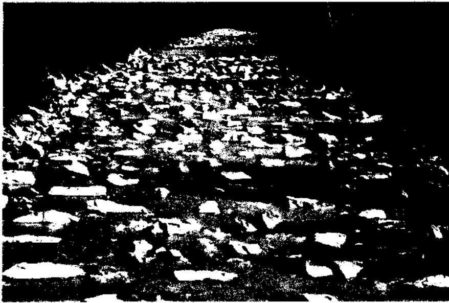
Fig.2.6a Unstructured block ramp application study on Landquart river (Janisch and Weichert, 2006)
