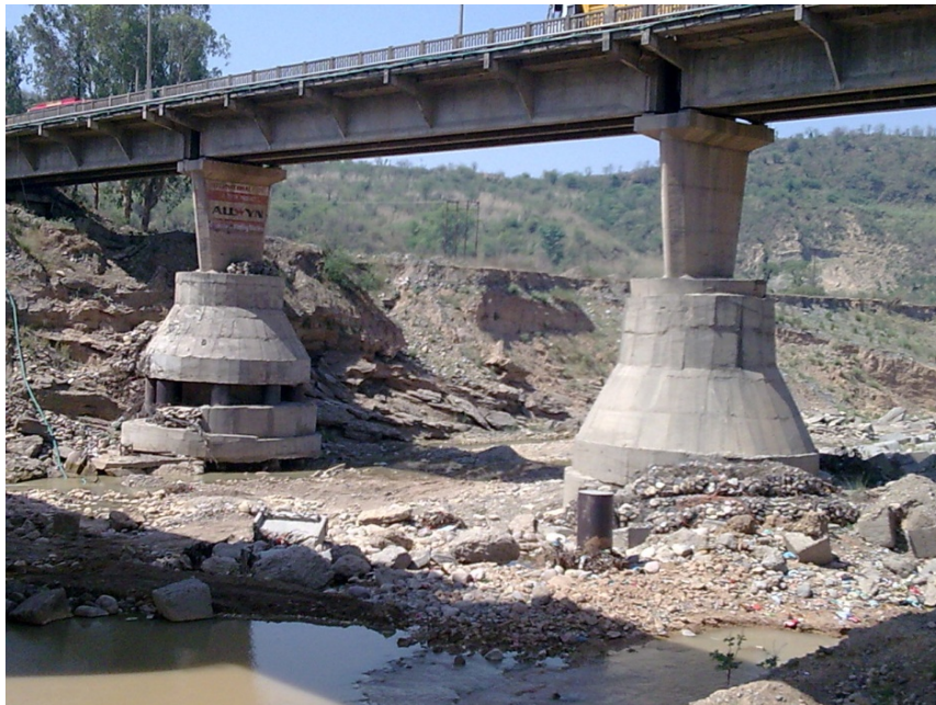
FIG. 1.1 Excessive scouring around footing of old bridge on river Chakki, Pathankot, Punjab
