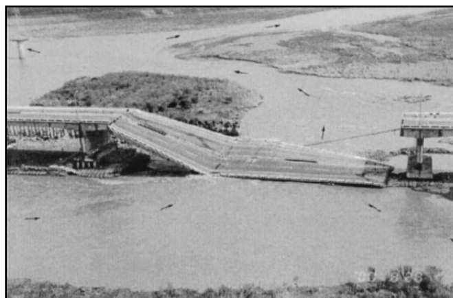
FIG 2.4 Failure of Kaoping Bridge, Taiwan, due to Combination of General and Local Scour (Chiew et al. 2004)
