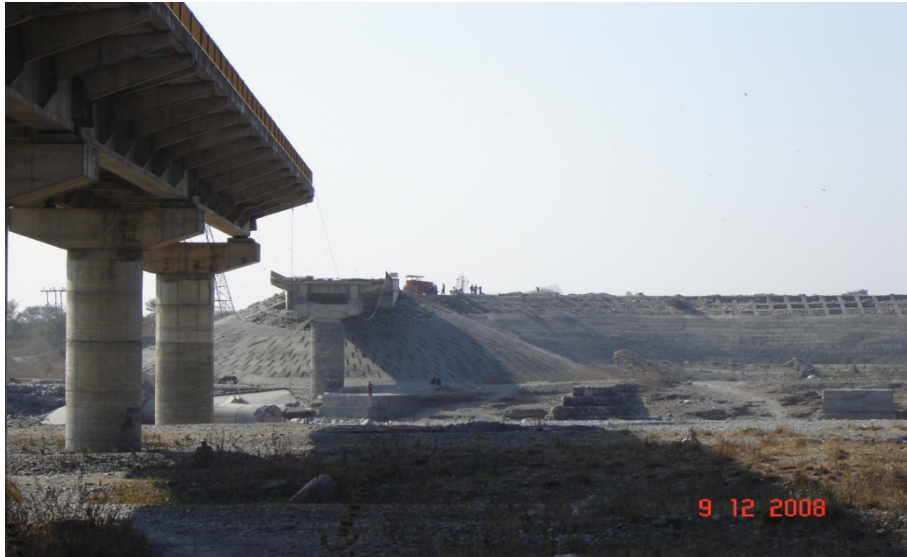
FIG. 1.4 Failure of Bridge on River Gola at Haldwani, Uttarakhand (2008)
