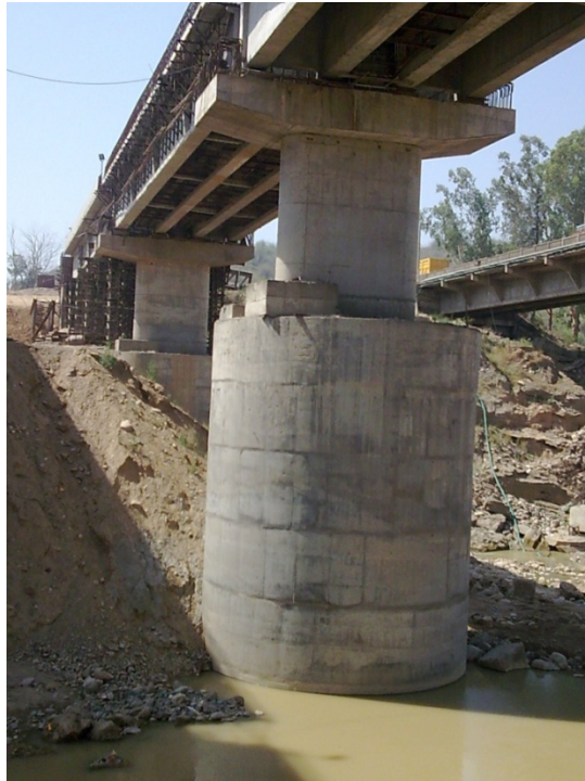
FIG. 1.2 Excessive scouring around footing of new bridge on river Chakki, Pathankot, Punjab
