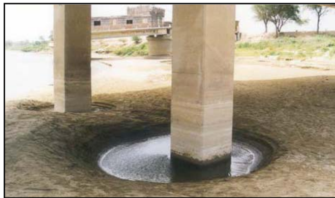
FIG 2.3 Photograph of Local Scour at Rectangular Piers ( www.pepevasquez.com )
