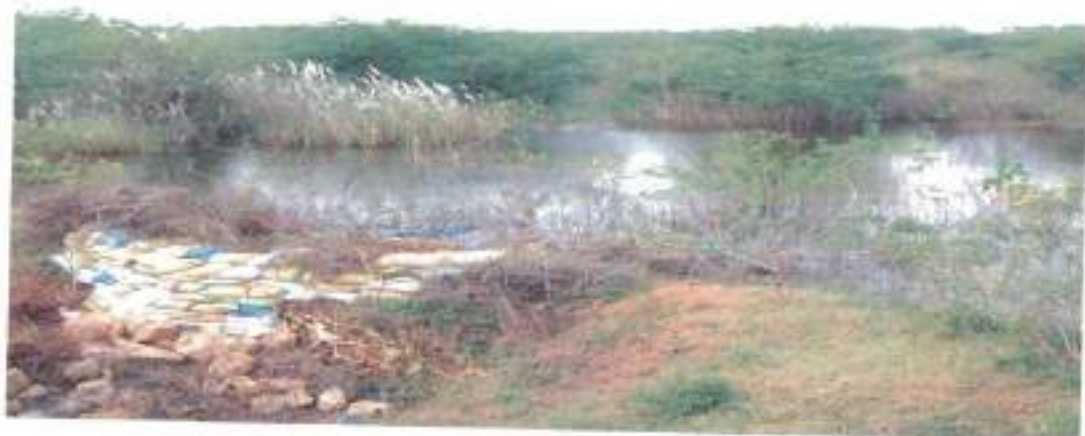
Photograph 4.3 Sand Bag Packing to Arrest the Breach at Ponpadi Tank during December 2008
