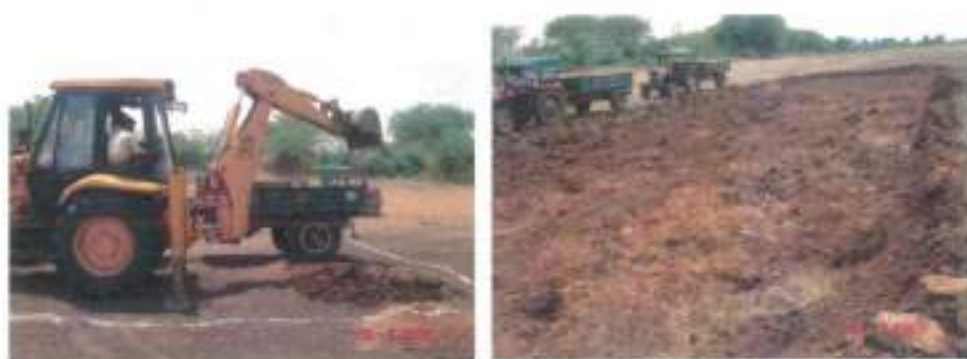
Photograph 5.1 Partial De-silting at Sengulam Tank
