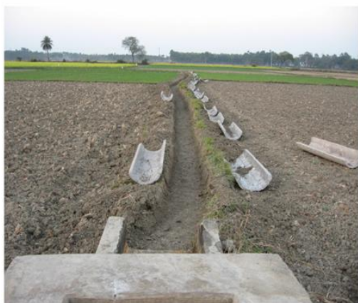
Fig.21 Channels under the process of construction
