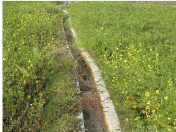
Fig.16 Completed bamboo-reinforced concrete channels
