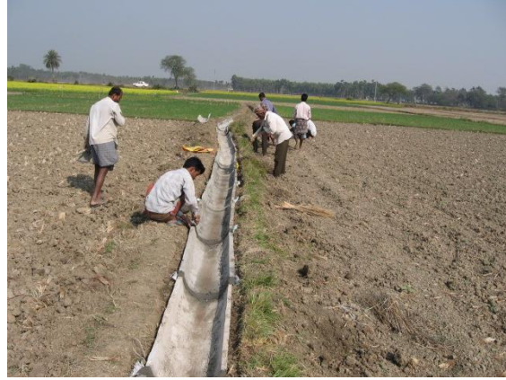
Fig.16 Completed bamboo-reinforced concrete channels
