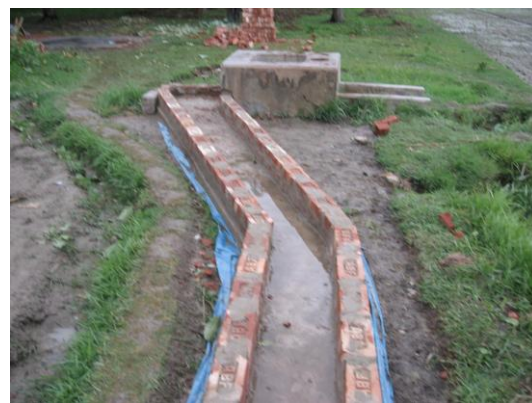
Fig. 11 Brick bats used in brick channels Fig.12 Brick channel in progress
