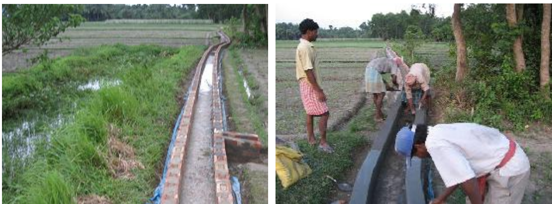
Fig. 25 Brick channels are in progress
