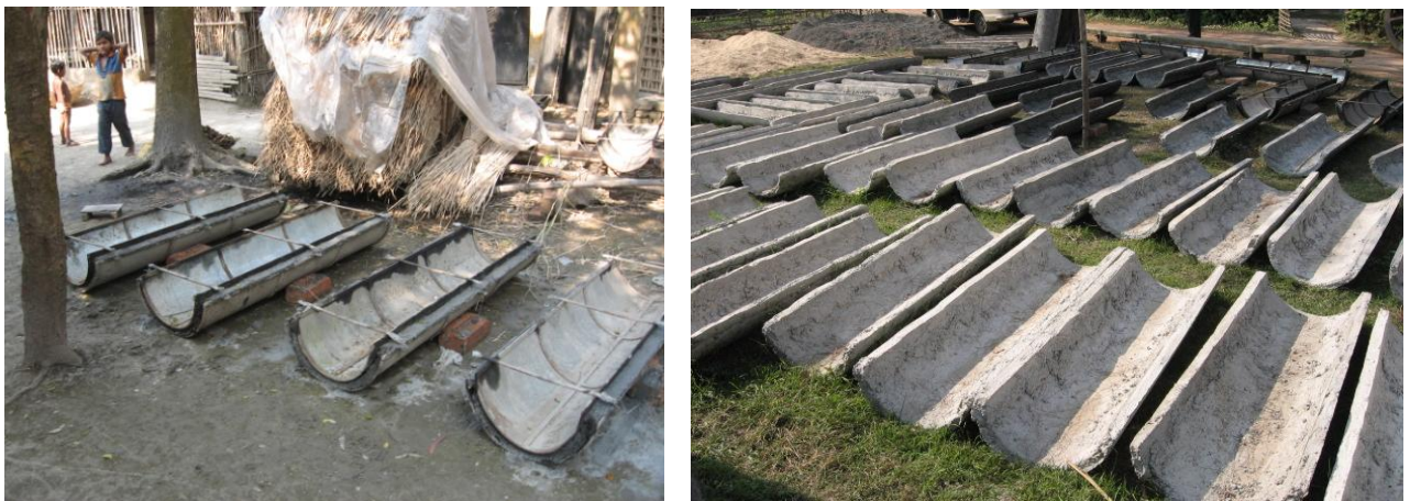
Fig. 4 Progress of casting the half round Fig.5 Concrete sections is ready for use bamboo- reinforced precast section
