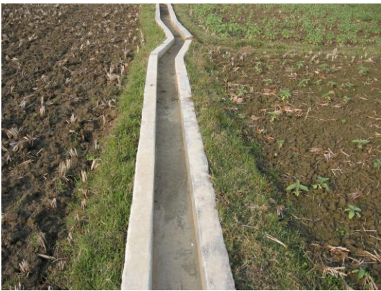
Fig.16 Completed bamboo-reinforced concrete channels
