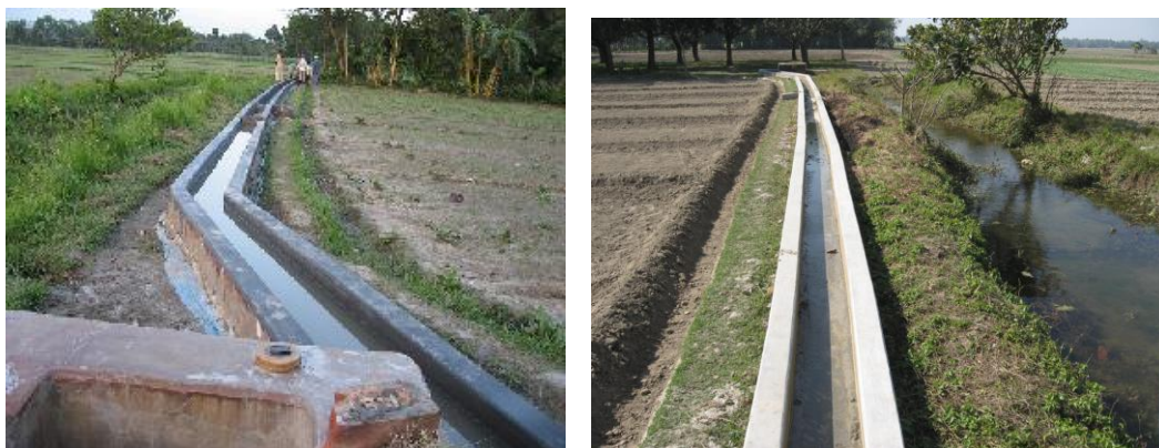
Fig. 26 Complete brick channels
