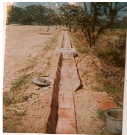
Fig.10 Laying of the earthen tiles in the channels
