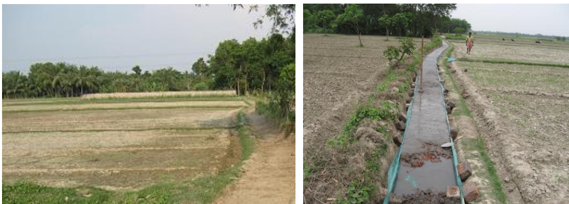
Fig. 23 Channel bed preparation of for brick Fig.24 Concreted bed for brick channel
