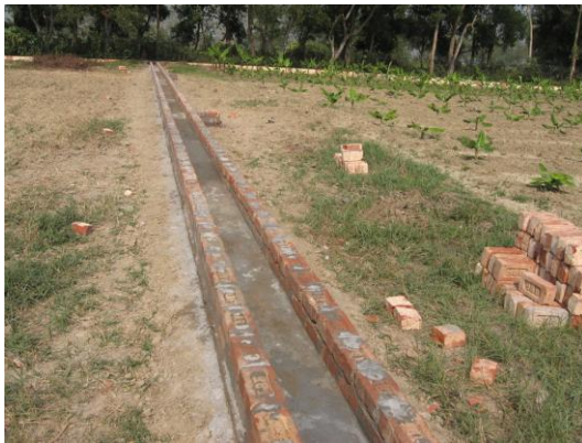
Fig. 40 Brick channel in progress
