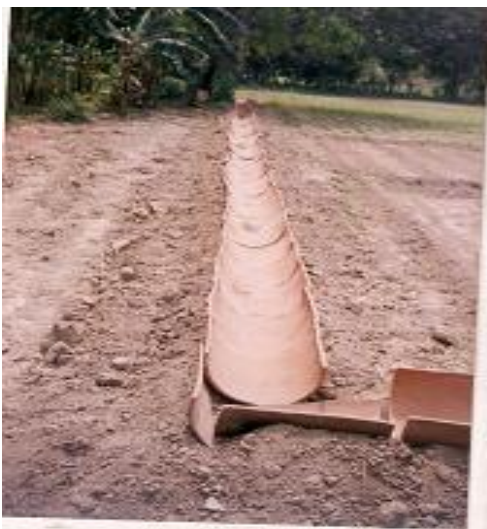
Fig.10 Laying of the earthen tiles in the channels
