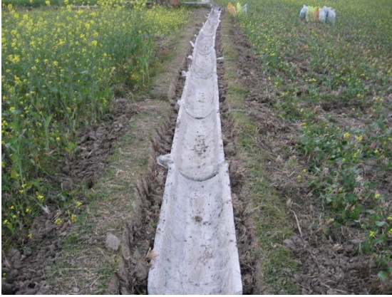
Fig.16 Completed bamboo-reinforced concrete channels
