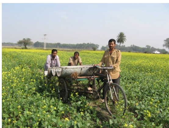
Fig. 14 Concrete sections are carried in the Site through van-rickshaw
