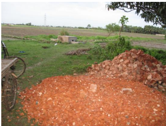
Fig. 11 Brick bats used in brick channels Fig.12 Brick channel in progress
