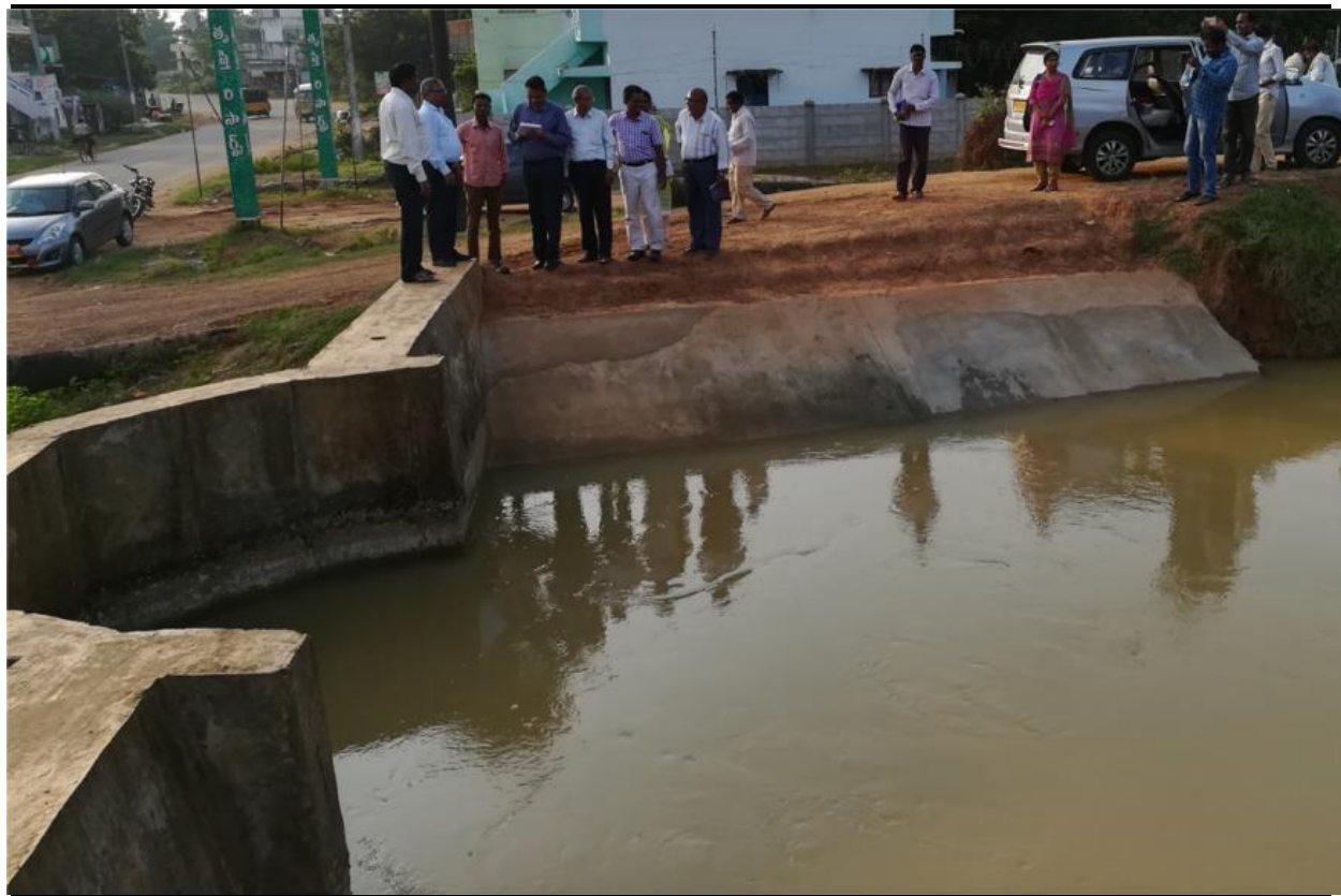
Canal Syphon On Rajam Branch Canal of Thotapally Project
