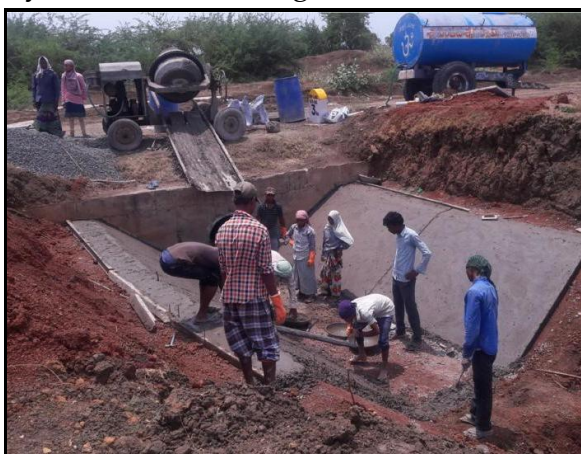
Ongoing lining work on Canals of Gundlakamma Project
