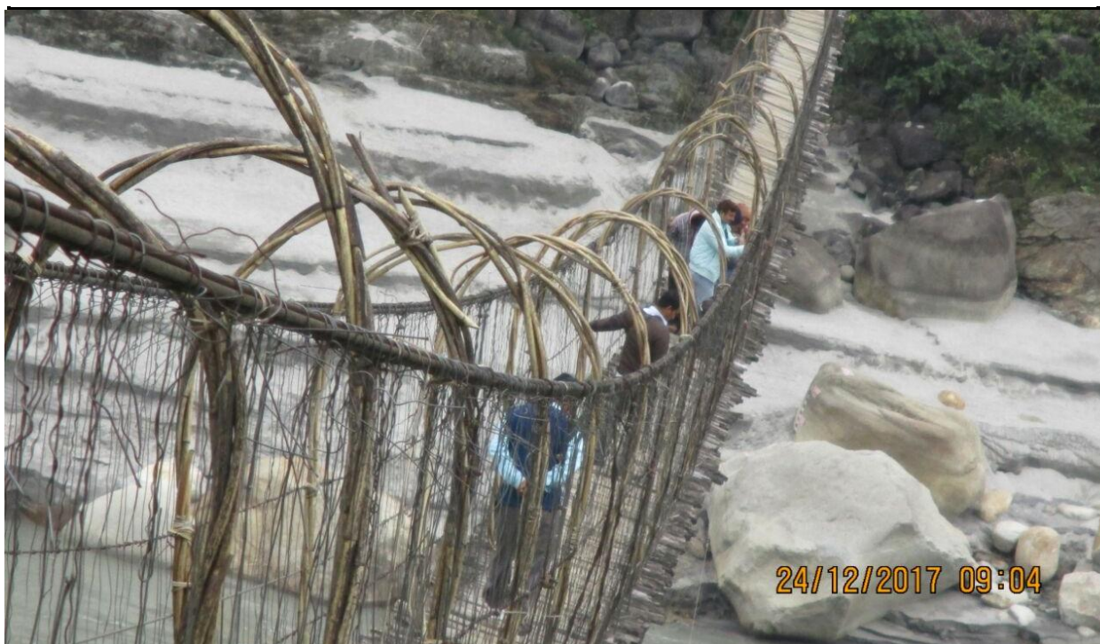
Gauge and Discharge observation through cable bridge in hilly region.
