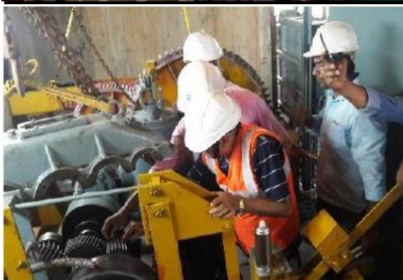
Inspection of gate hoists at Maithon and Panchet Dams
